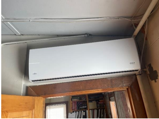
Cooling – Ductless Fan Coil Unit
