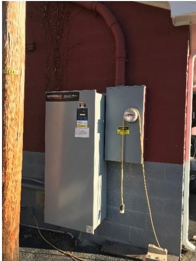
Automatic Transfer Switch
