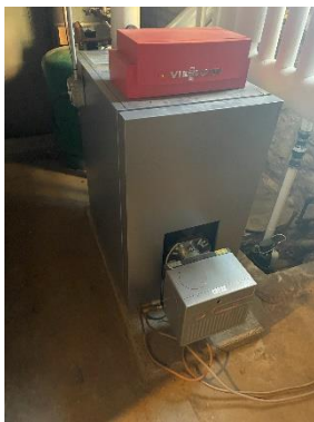
Hot Water Boiler
