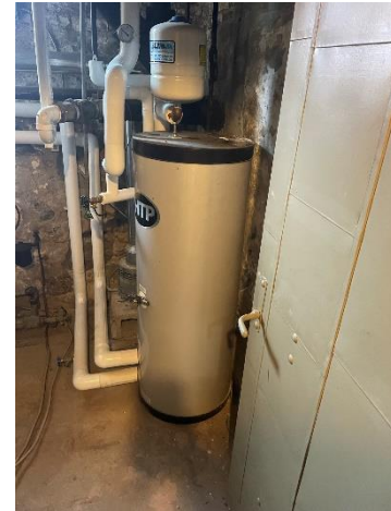
Indirect Hot Water Heater
