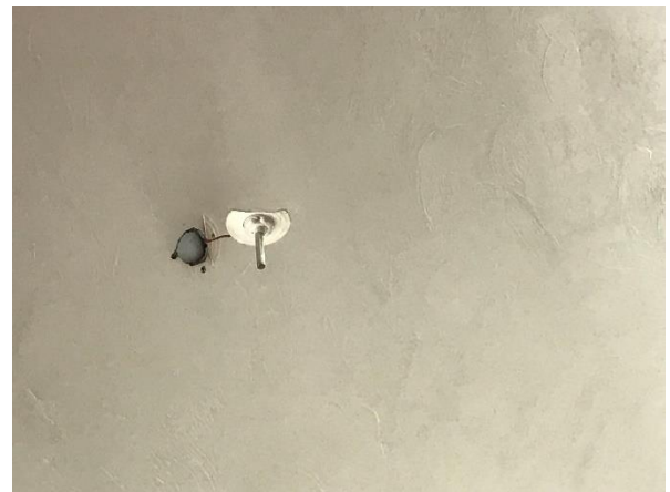
Broken Heat Detector
