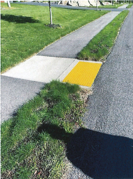
Sidewalks and handicap ramp
