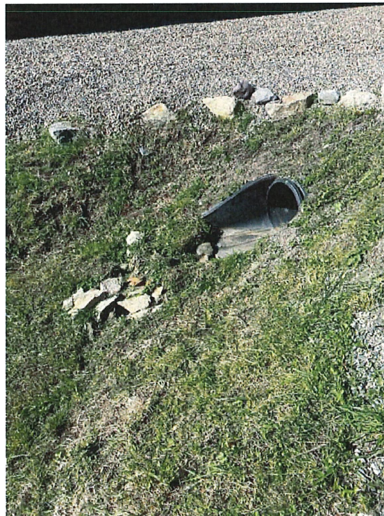
Rip-rap pad at discharge to sediment forebay
