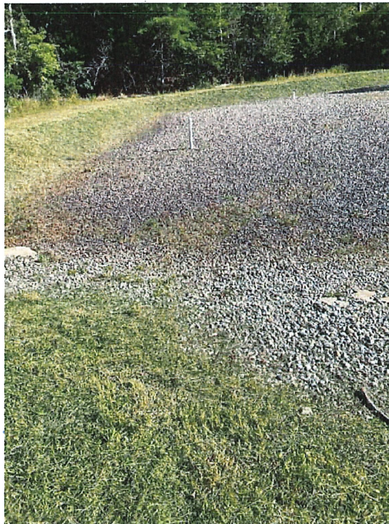
Bottom of infiltration basin
