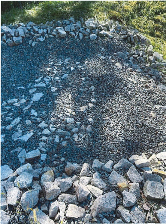
Overflow weir from infiltration basin
