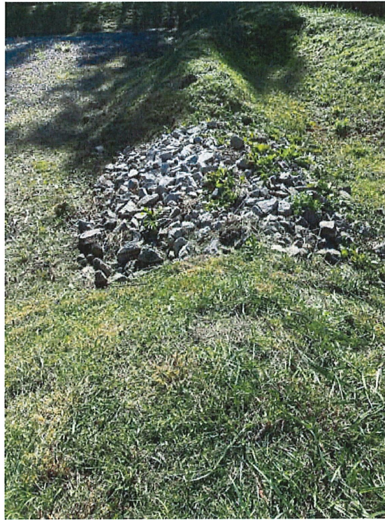
Overflow from sediment forebay
