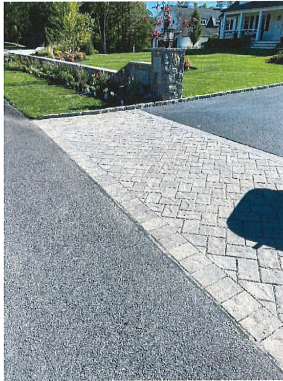
Stamped concrete at driveway
