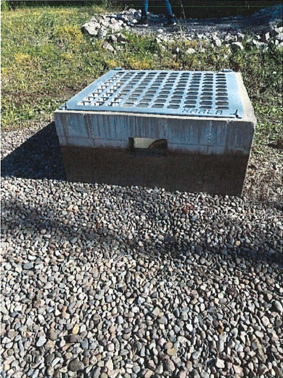
Outlet control structure from infiltration basin
