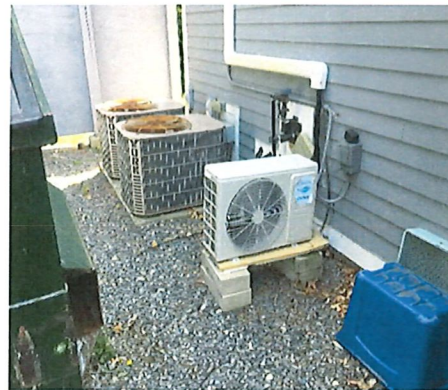
Existing Outdoor Condensing Units (Ductless AC unit)
