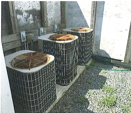
Existing Outdoor Condensing Units
