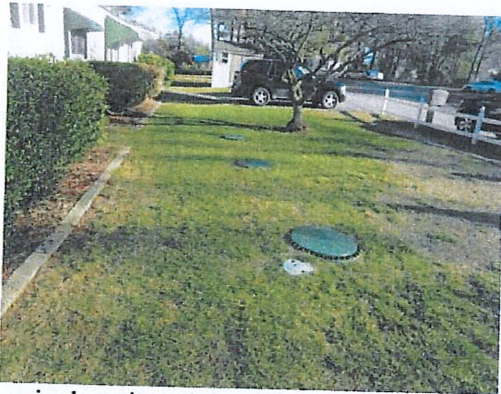
Repaired septic and covers
