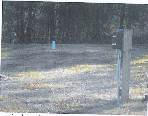
Repaired septic system
