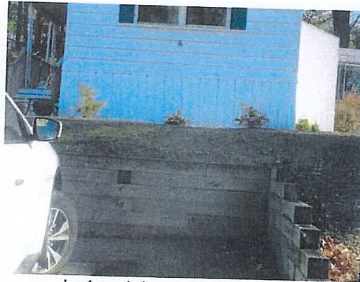
repaired retaining wall
