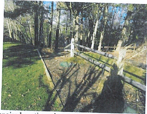
Repaired septic and covers
