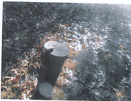
typical artesian well, exposed wires
