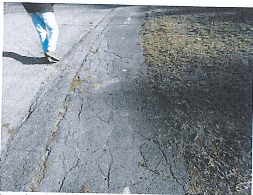
Deteriorated sidewalk
