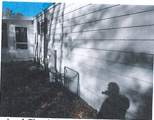
Replaced. Electrical meter panel
