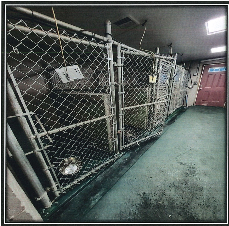
Strip concrete floors of old finish, sand and prepare concrete for a new Epoxy floor refinishing.
