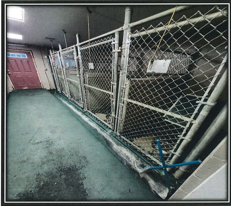
Strip concrete floors of old finish, sand and prepare concrete for a new Epoxy floor refinishing.
