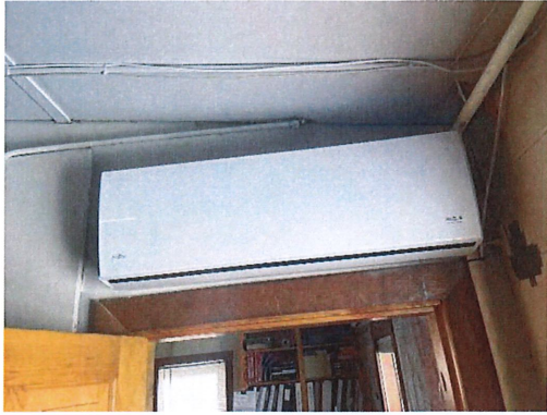
Cooling – Ductless Fan Coil Unit
