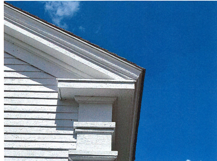
4 FASCIA/ RAKE CONDITION
