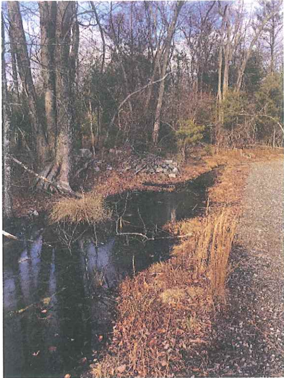
Standing water west of Infiltration Basin
