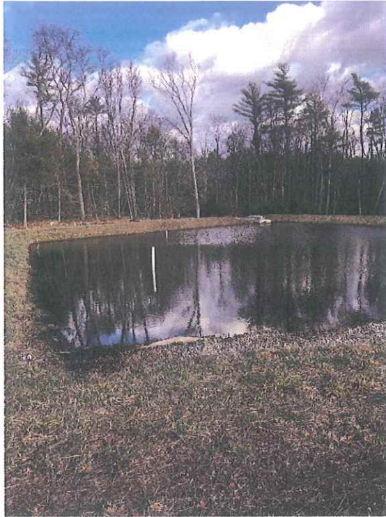
Standing water in Infiltration Basin
