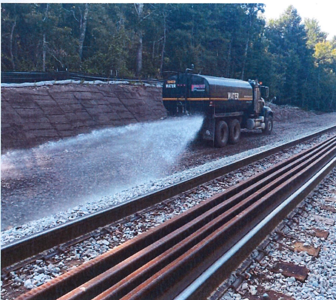
Dust control Cotley Street right of way
