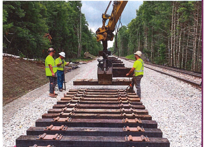
Setting ties on the right of way
