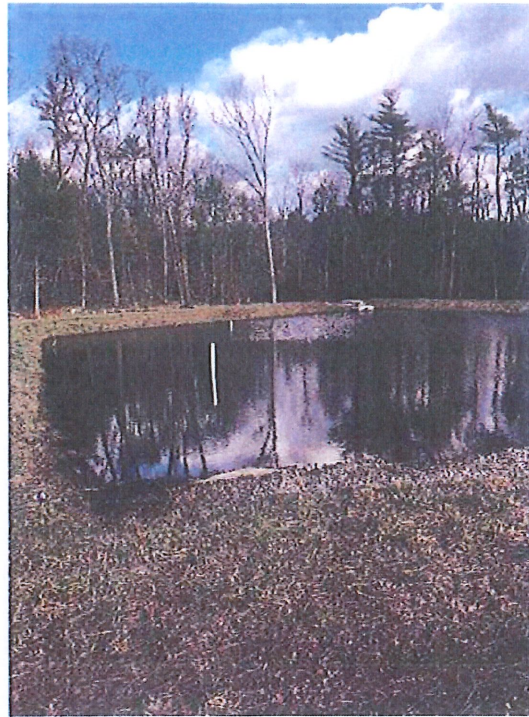
Standing water in Infiltration Basin
