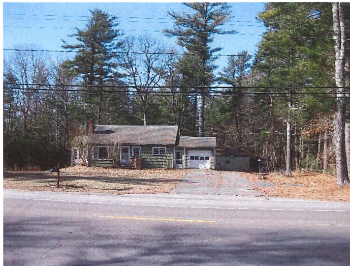
Proposed subdivision roadway location at Bedford Street; characterization of existing home
